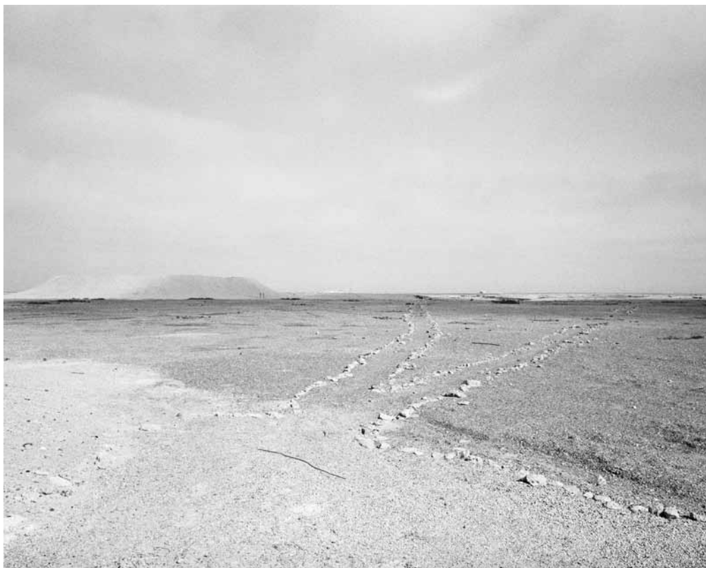
SAM missile bunkers, Cuban base, Namibe, 2010
