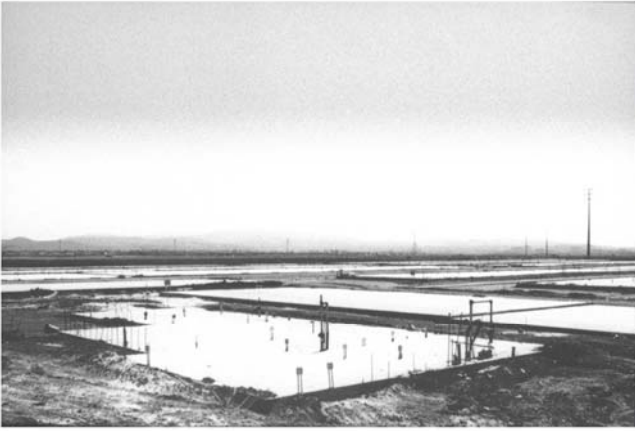
032 Baltz Lewis_14_NIP_Foundation Construction_Many Warehouses_2891 Kelvin_Irvine.jpg
